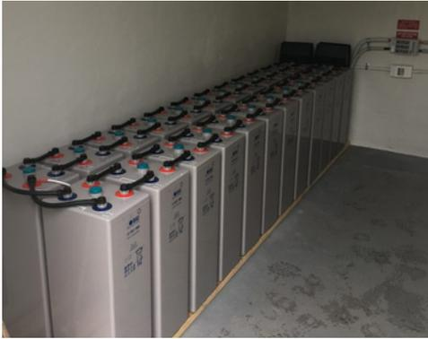
Another thing to understand is diminishing capacity: All batteries, irrespective of their chemistry will lose storage capacity (kWh) over time. The more energy that goes through a battery per day, the faster the capacity will diminish. A larger battery (relative to your usage) will provide for you longer than a small battery.
