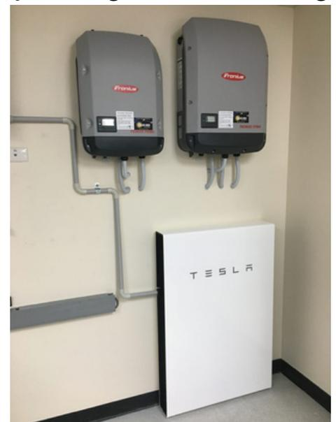
A secondary function of some battery units is to provide back-up power during a grid outage. Contrary to popular belief, not all battery systems can provide power during an outage. Some have only limited capability (eg to run your fridge or lights).
